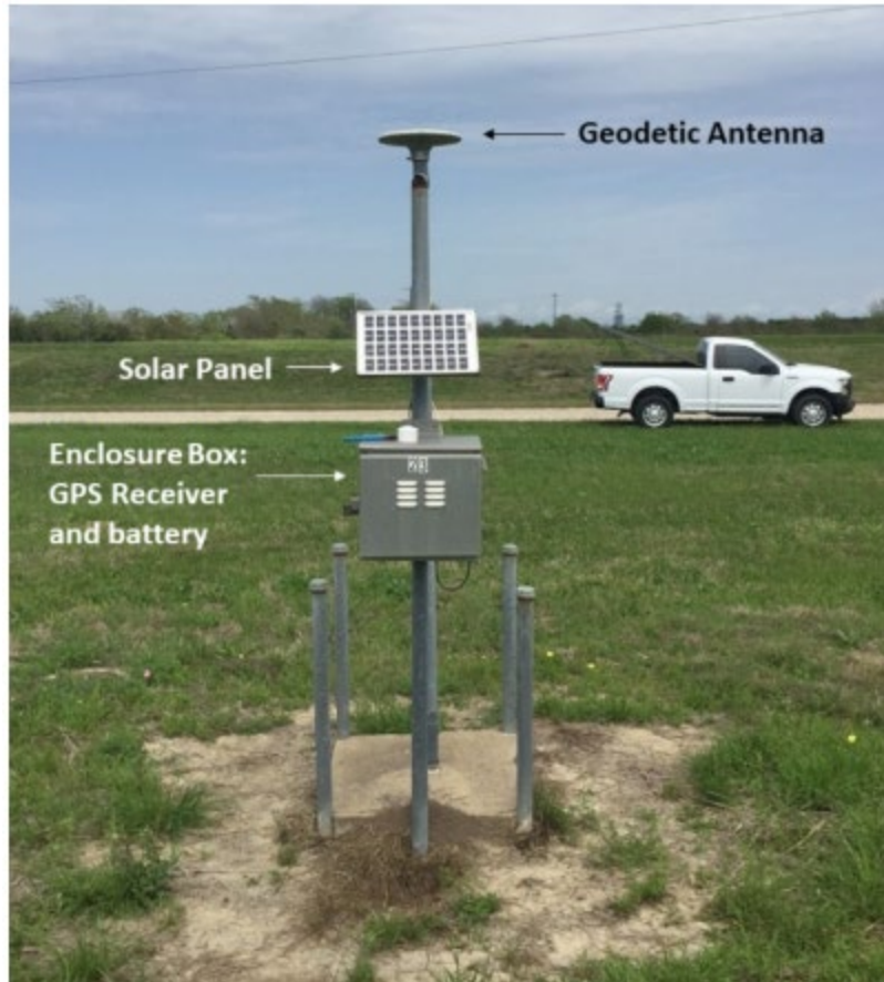
Figure 4-6 Example of a complete subsidence monitoring station with all geodetic instrumentation and power supply equipment installed.
