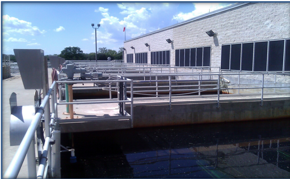
Figure 2: Victoria WTP Filters
