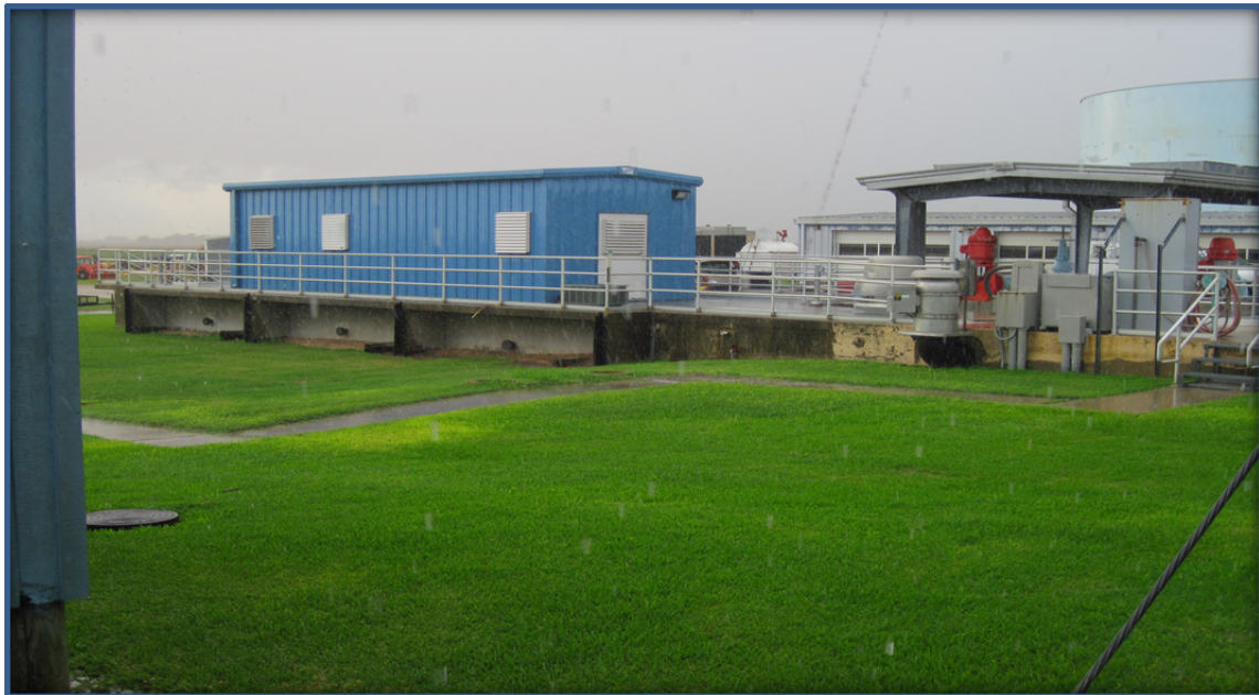
Figure 7: PLWTP Filters and Transfer Pumps
