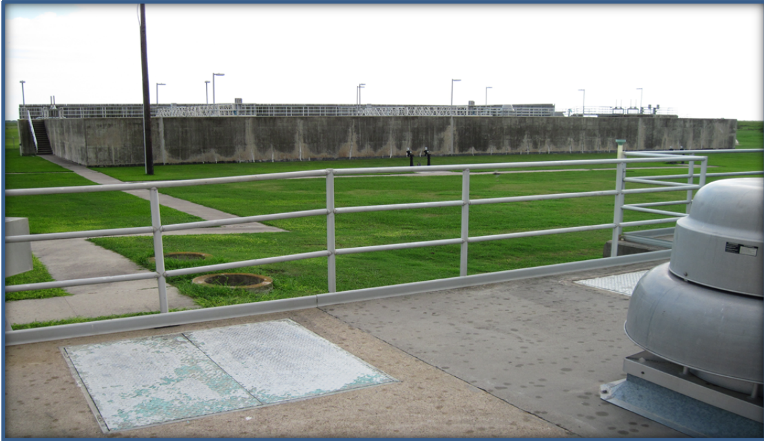
Figure 6: PLWTP Settling Basins
