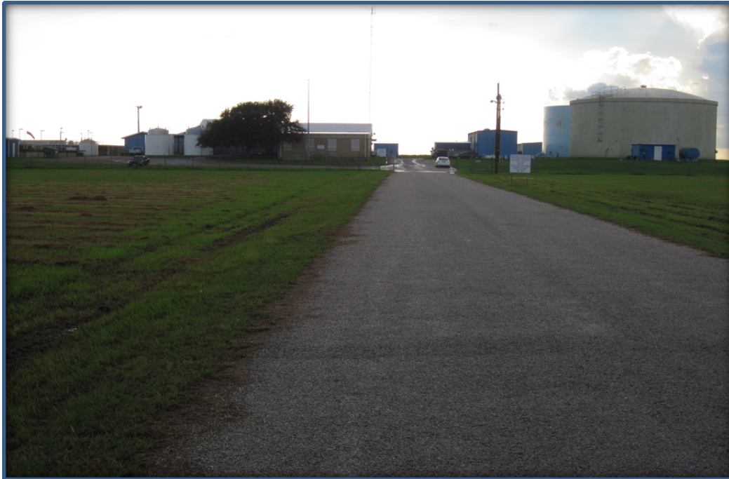
Figure 5: Port Lavaca WTP Entrance
