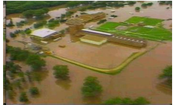
Des Moines Water Works, Iowa – 100 MGD WTP Before and After 1993 Flood
